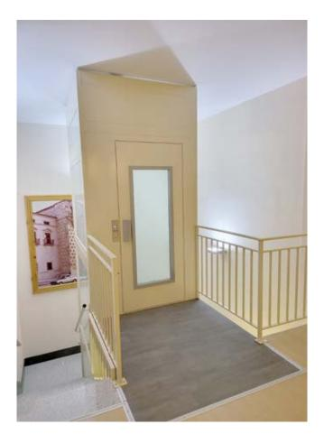
The **ECO-EXCEL** residential lift model is a hydraulic lift that has all the features of a conventional lift.
